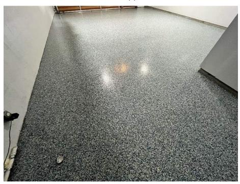
In addition to their physical strength, epoxy coatings create a protective barrier that helps prevent damage from chemicals, oil spills, and stains. The impermeable nature of epoxy makes it resistant to various substances that may be encountered in a typical garage environment. Whether you accidentally spill motor oil or drop harsh chemicals on your floor, an epoxy coating will provide a reliable shield against potential damage.
